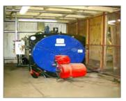
Methane gas is produced to run the engine that produces the electricity, with an additional pipe line installed to the mill where the gas is used to run a boiler; this in turn produces the steam for use in the production process. The waste product from the digester is then pumped through a pasteurizing unit into a holding tank where farmers collect the product with tractors and tankers to spray back onto the fields as fertilizer.
